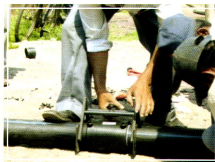
Jointing of Pipes Electro fusion coupler
